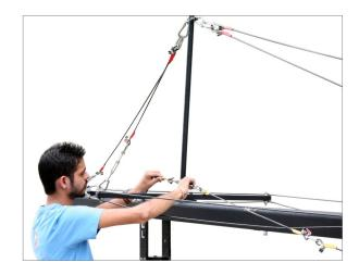
Attach the Pan Tilt Head with the Jib.
